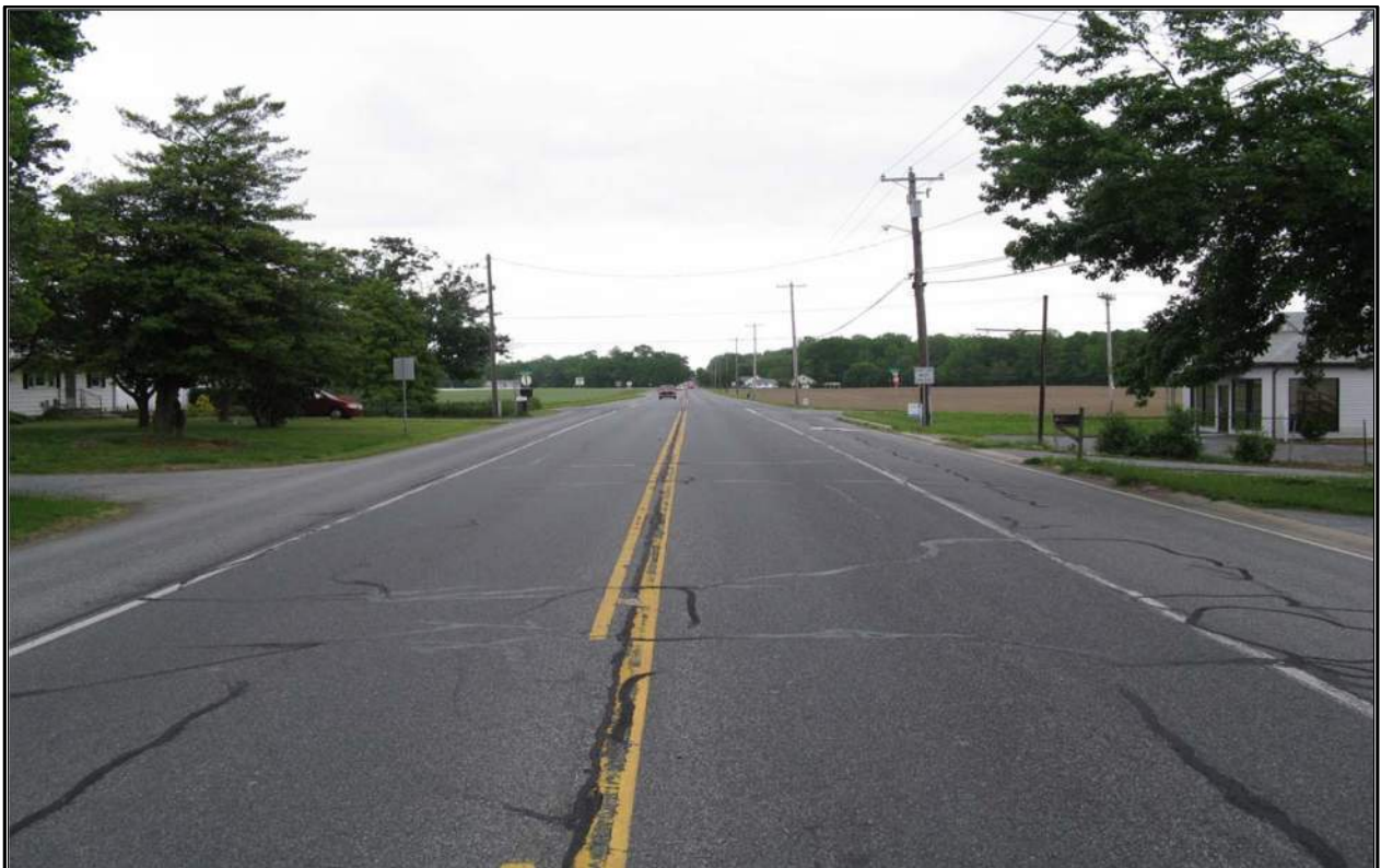
2) DE Route 8 looking East toward Chestnut Grove Road / Nault Road
