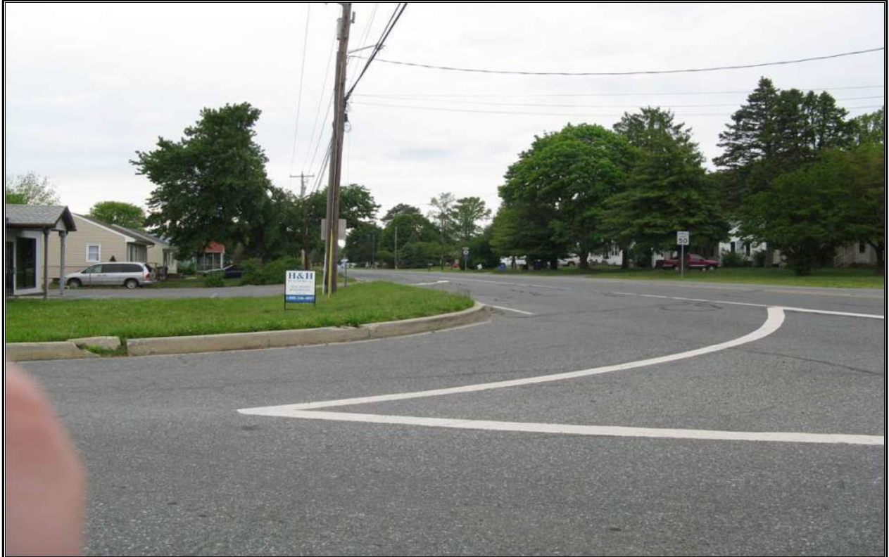
7) Northbound Nault Road Looking Left (West)
